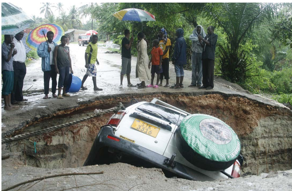
Figure 11: Road destruction by floods at Tandale Mtogole, 2011
